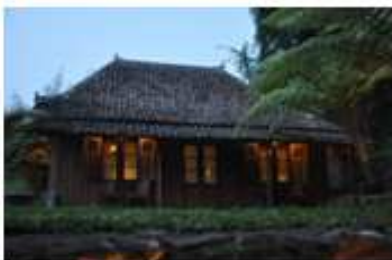
Picture 4.14. Front façade (Source: Susy Budi Astuti)
