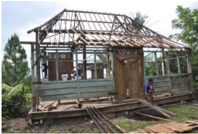
Picture 4.12. Front façade (Source: Susy Budi Astuti)
