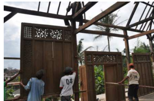
Picture 4.11. Process of surface assembling (gebyok) (Source: Susy Budi Astuti)
